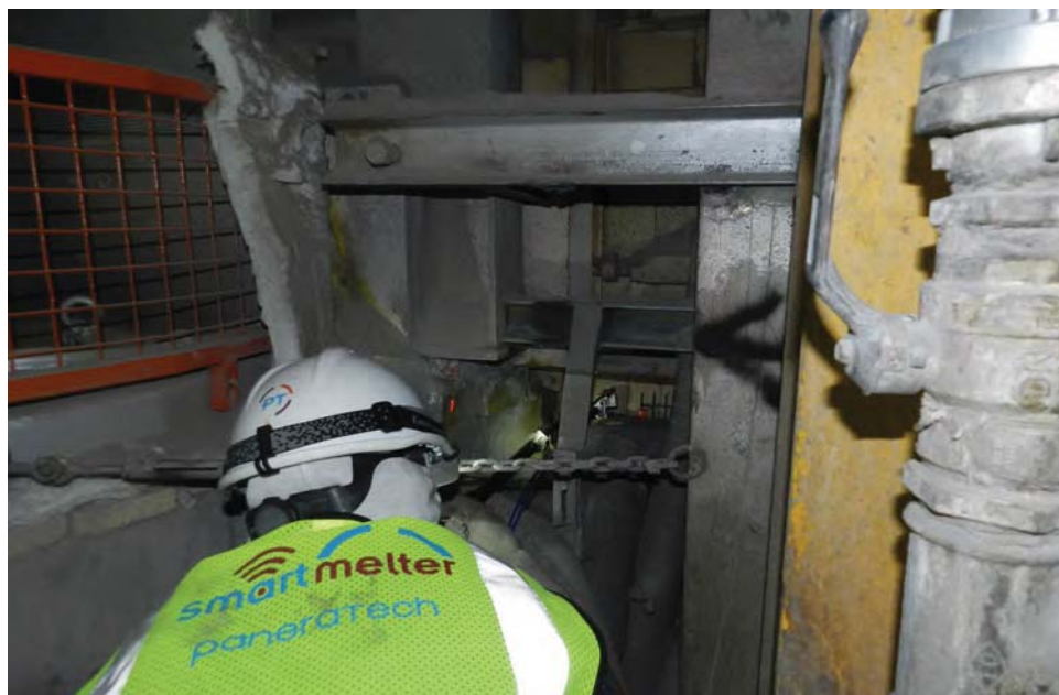
Figure 5 PaneraTech team member taking measurements on the furnace
